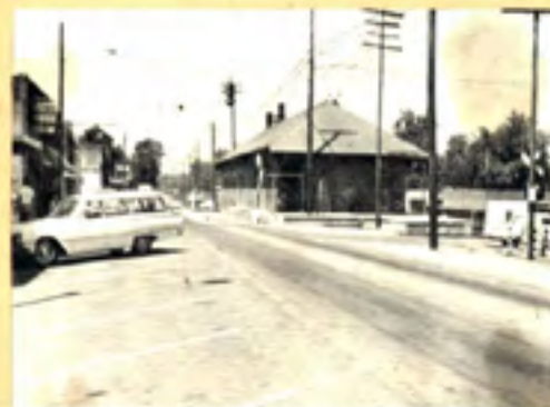
Railroad Station showing the date 1867 over the doorway. The first station was destroyed in the Battle of Jonesboro.
