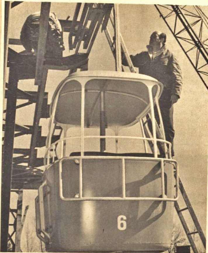
ALFRED BIGLER, A SWISS ENGINEER makes final adjustments on one of the gondolas of the Six Flags Over Georgia Astrolift. The Astrolift, will ride guests snugly 82 feet in the air from a cable track supported by three 90-foot towers.
