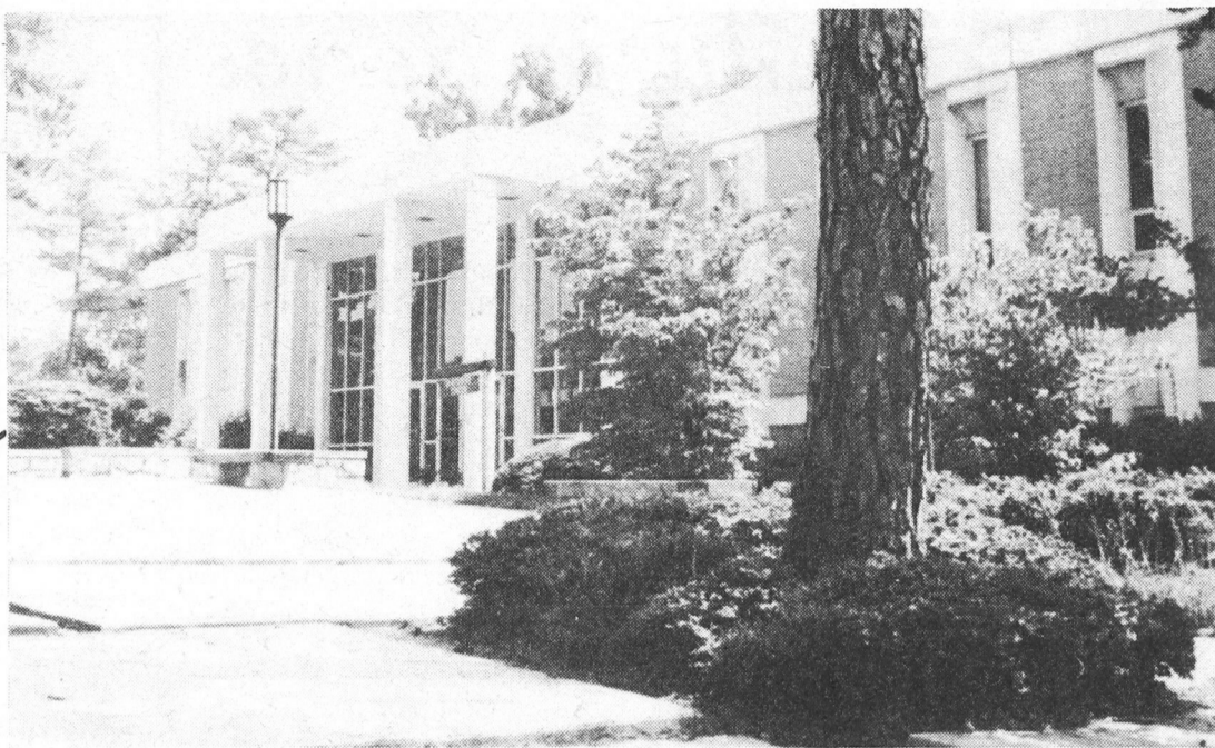
The D-Student Center Building is home to the Counseling Center (D-208) and the Student Lounge (including the offices of Student Government and The Bent Tree ). Vo-Tech and Business labs, faculty offices, and classrooms, along with the Public Safety Office, are on the upper level. The lower level features the Dental Hygiene Clinic, Dining Hall, and the College's Bookstore.
