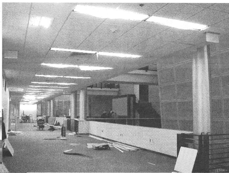
This is the second floor corridor with classrooms to the left.
