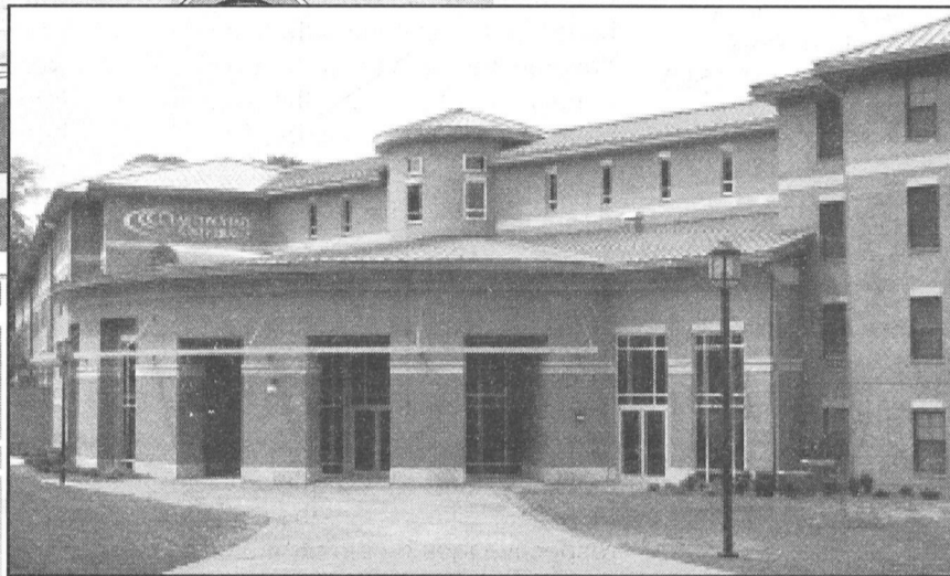
Laker Hall, Clayton State's New Dormitory
