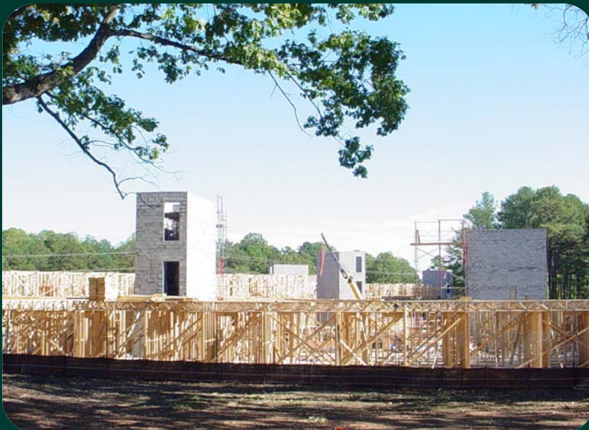
Construction on the new Student Housing facility. Photo taken on October 27, 2007
