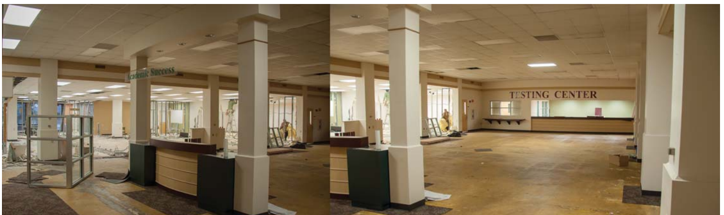
Library Renovation Progress
